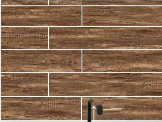
**Step 9:** Use a hammer and pull bar to lock long edges of planks on the final row.
